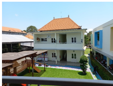
Gambar 2 Damar Bali School (Sumber: Penulis, 2023)
