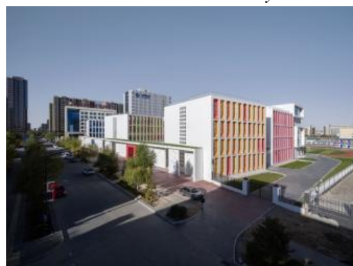
Gambar 8 Fasad Bangunan Yulin Gaoxin No. 3 Primary School (Sumber: https://bit.ly/31dd8Ib , 2021)
